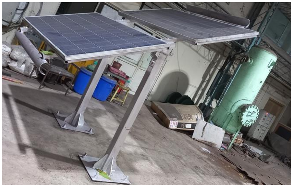
Figure 57: Final fabricated prototype of the solar PV support structures being installed at Ghoramara demo site.
