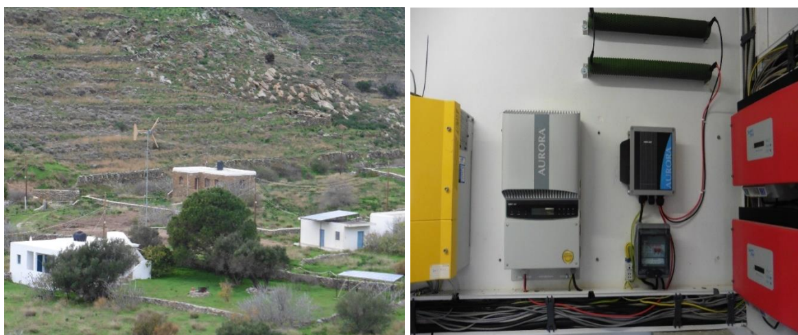
Figure 59: The LMSWT installed in the microgrid (left), Inverter, over-voltage protection and dump loads (right)
