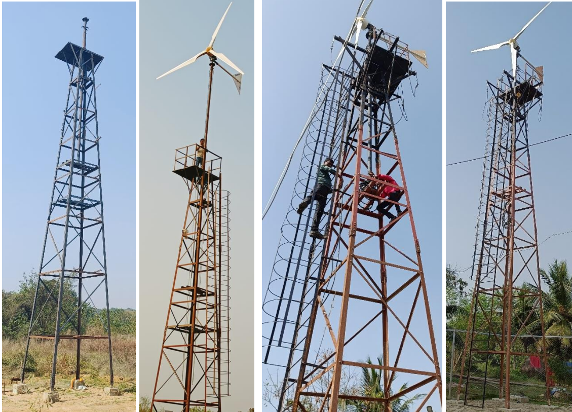
Figure 118 Installation of tower at testing at CSIR-CMERI & demo site, Ghoramara for power generation.
