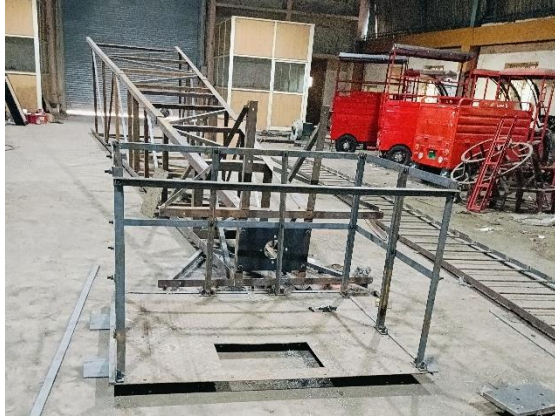
Figure 117 Making of foundation and fabrication of hybrid tower as the final drawings
