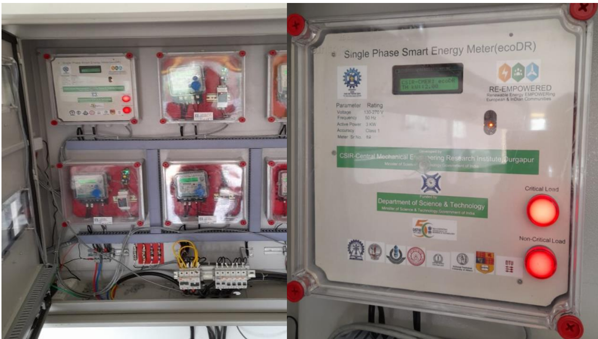
Figure 88 ecoDR (top left of the left picture) installed at Ghoramara and ecoDR monitoring load threshold data
