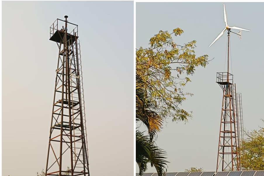
Figure 24. Installed hybrid wind turbine support at CSIR-CMERI for testing
