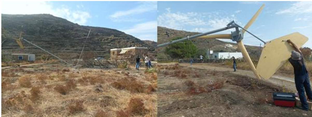
Figure 55: a) Locally manufactured SWT and tower lowered for maintenance, b) LMSWT being maintained by project partners and user community.
