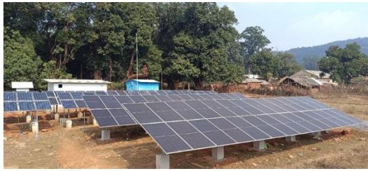
30 kWp new solar PV plant
