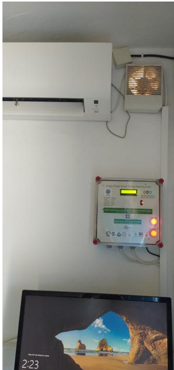
Figure 49: ecoDR deployment at Gaidouromantra control room. Interposed to HVAC power supply.
