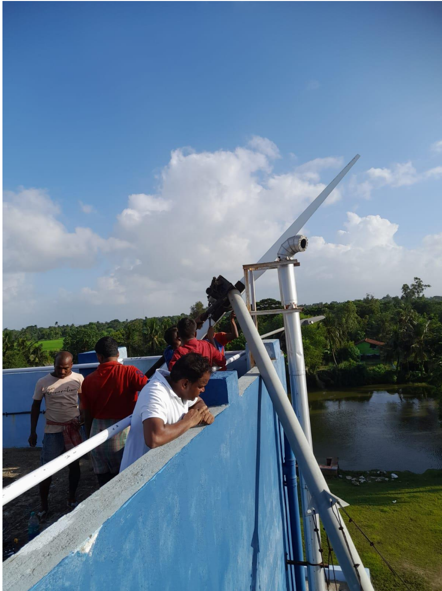
Figure 25: Decommissioning of pre-existing wind turbine support structure with the help of Ghoramara local people.
