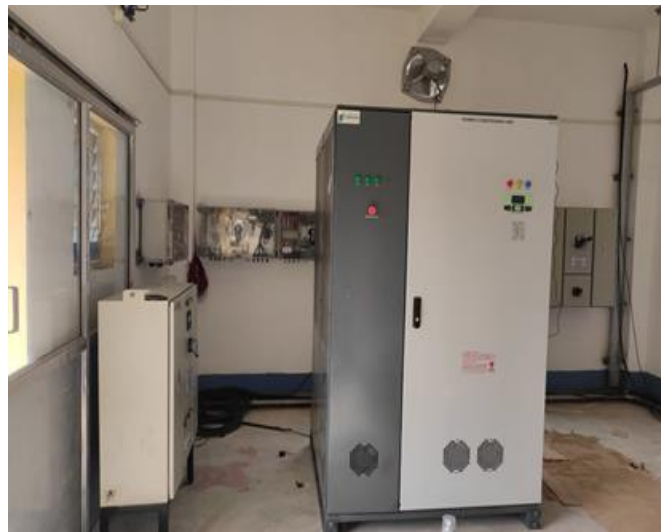
Figure 5: Inverter in Control room at Ghoramara
