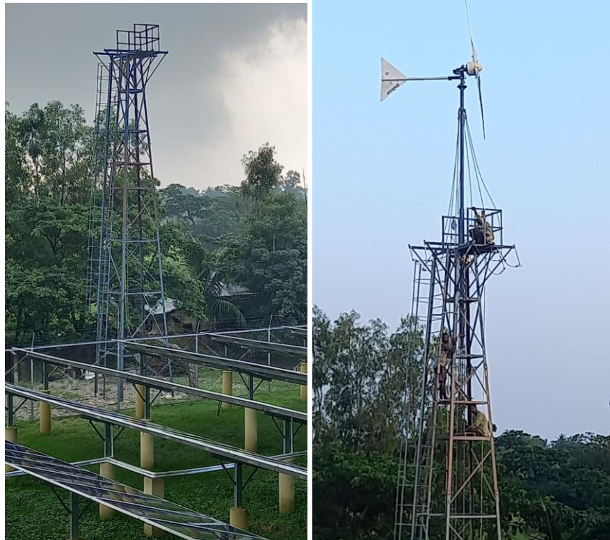
Figure. 25 Installation of hybrid support structure with wind turbine at Ghoramara site
