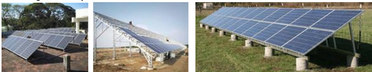
Figure 69: Conventional PV support structures
