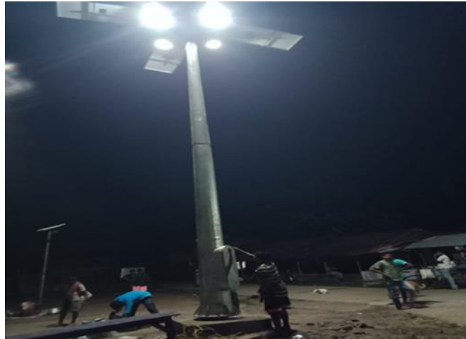
Figure 46. Solar Powered High-mast System at Ghoramara Island.
