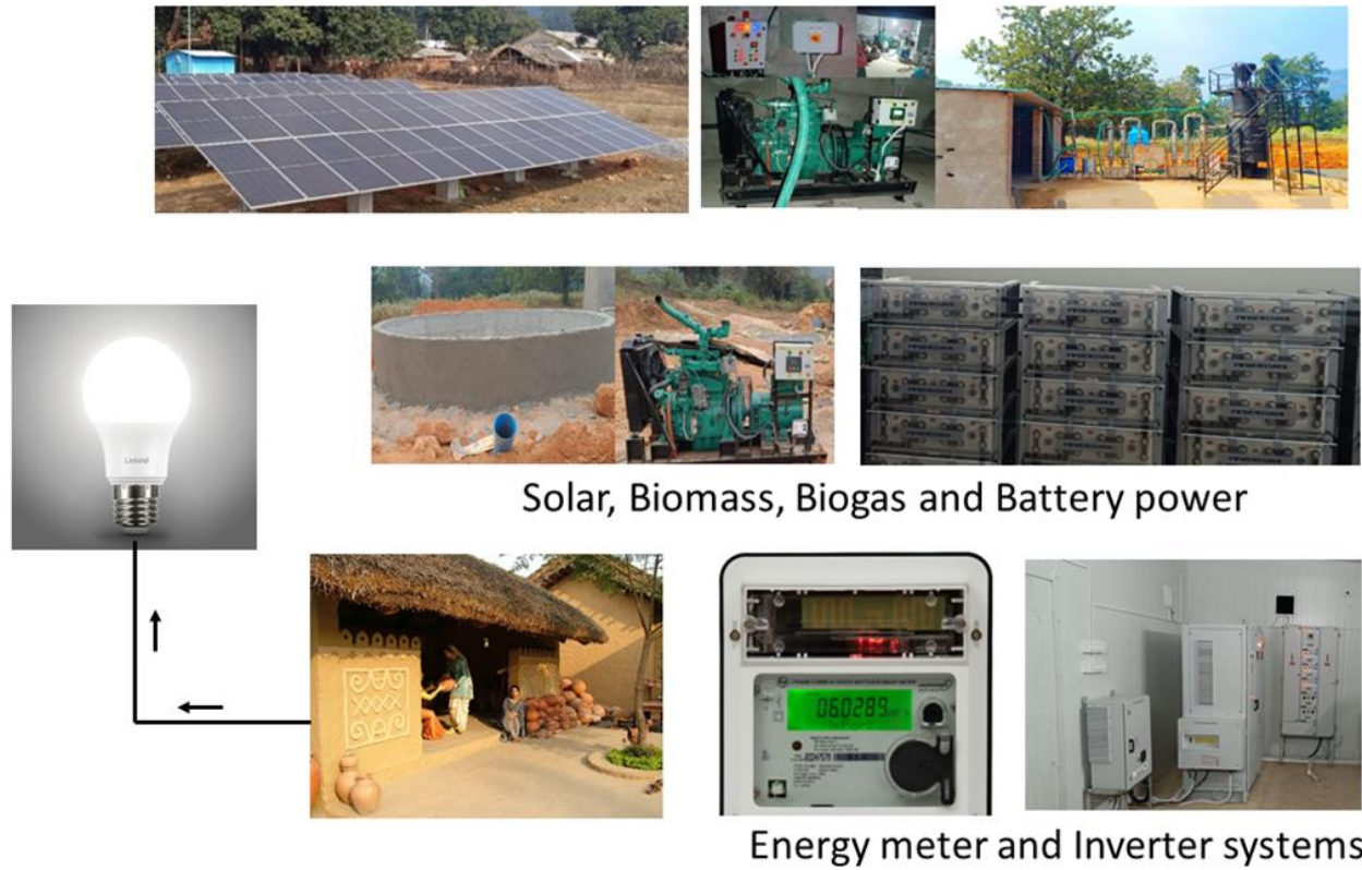
Figure 41. Different energy systems at Keonjhar microgrid Demo Site.
